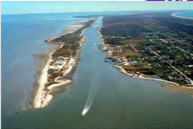
Galveston Bay. Photo courtesy U.S. Army Corps of Engineers/Flickr
