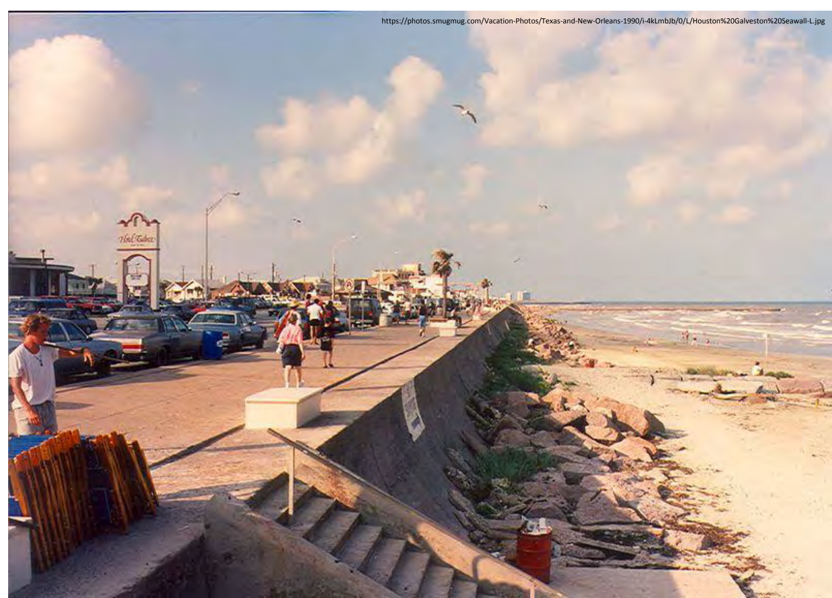
The Galveston Seawall was installed in the early 1900s to provide protection against storm surges. Storm surges will get larger as a result of SLR.
