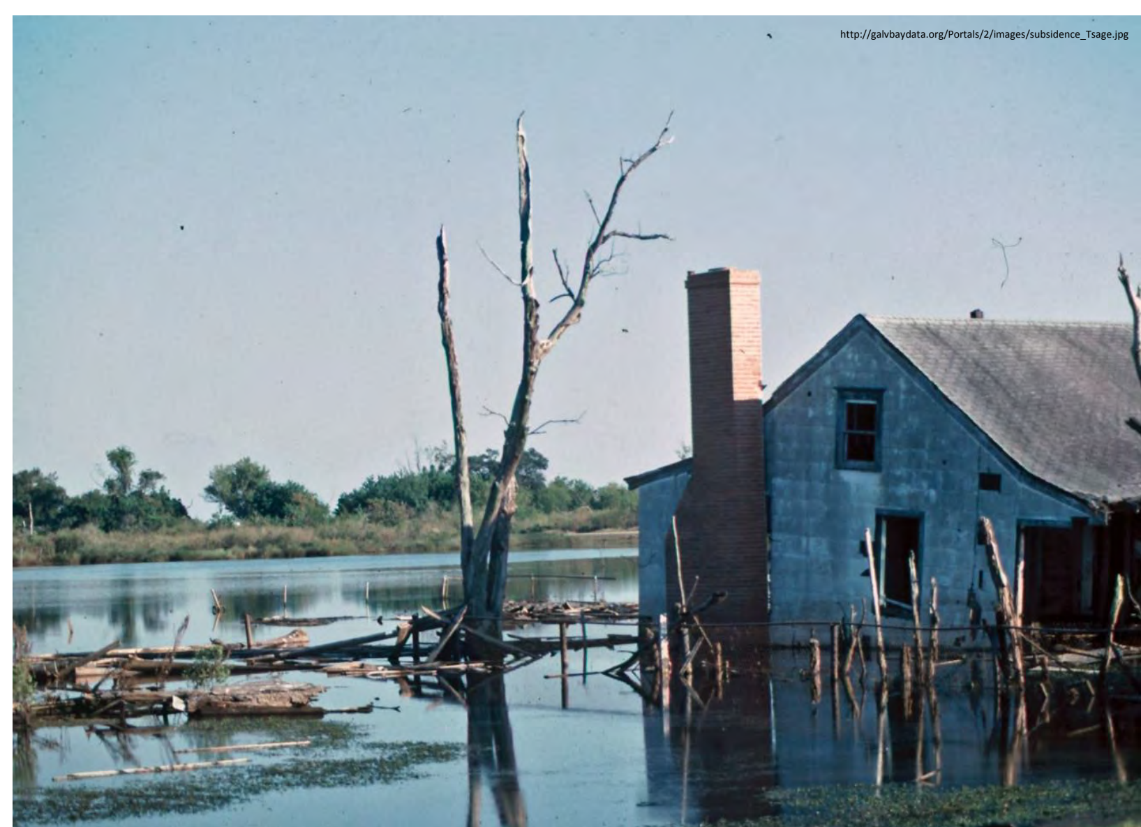
The Brownwood subdivision, located in Baytown, TX, was converted to the Eddie V. Gray Wetlands Education Center due to subsidence-caused inundation.
