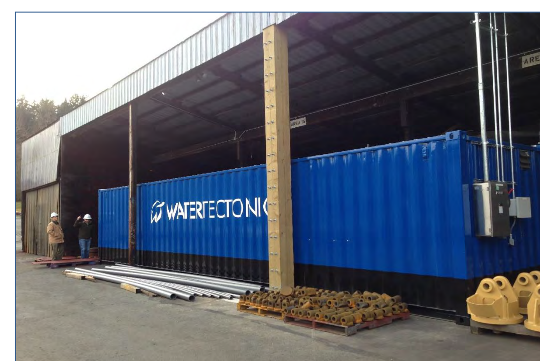
Picture 2. Industrial Facility Discharging to Puget Sound
