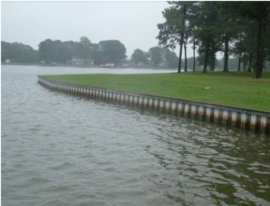
Talbot County, San Domingo Creek near St. Michaels
