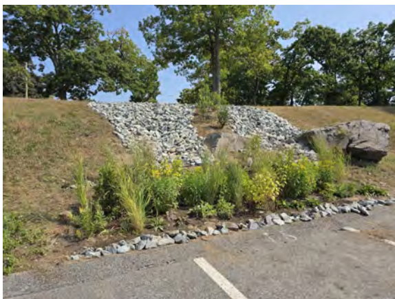
Photo (left) of riprap swales and rain garden at Boys & Girls Club of Pawtucket courtesy of GWRI and (right) rain garden at the Providence Journal property courtesy of WRWC.
