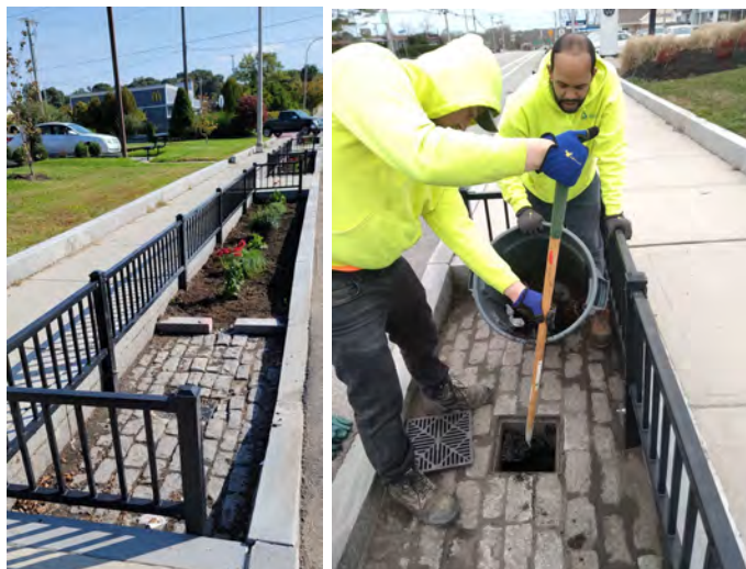
Photos of Old Tower Hill Road bioswales and maintenance courtesy of GWRI.
