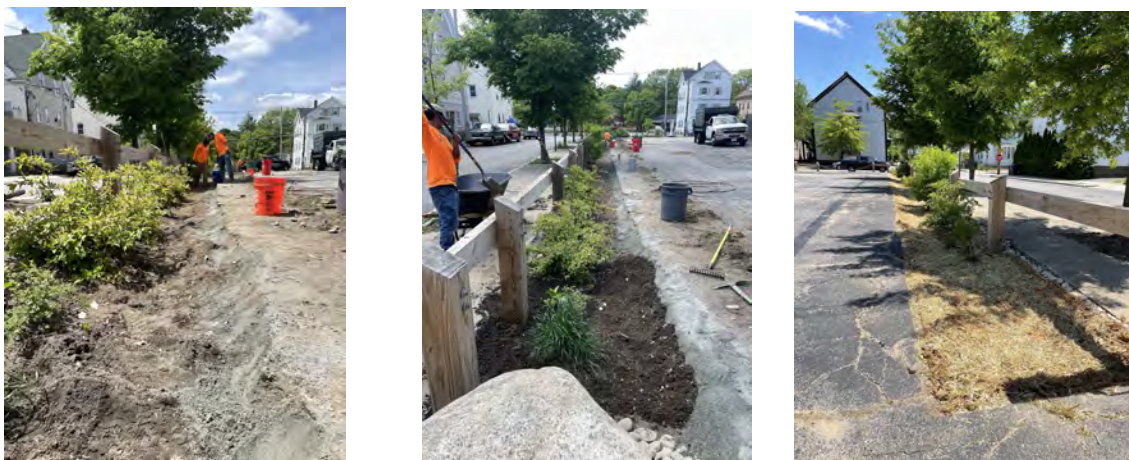
Damaged swales (above) at Puerta del Refugio Church before WRWC repairs (below). Photos courtesy of WRWC.
