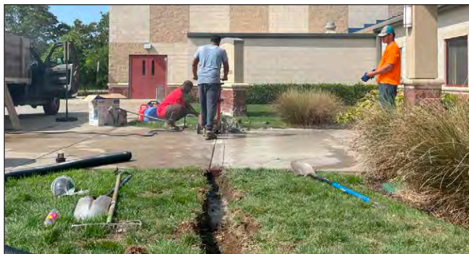
Dry well and linear drain install at area
