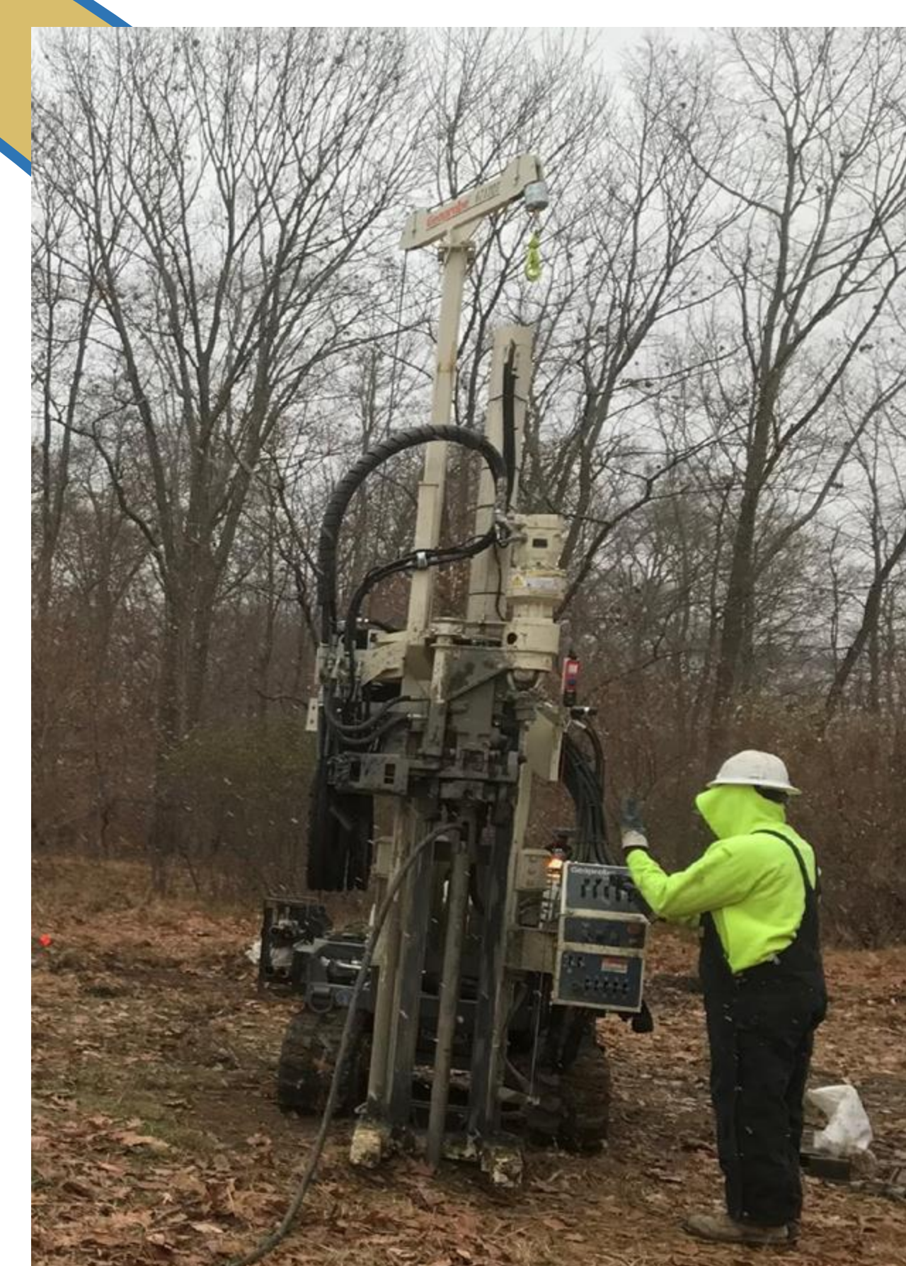
Direct push drill rig installing temporary injection point
