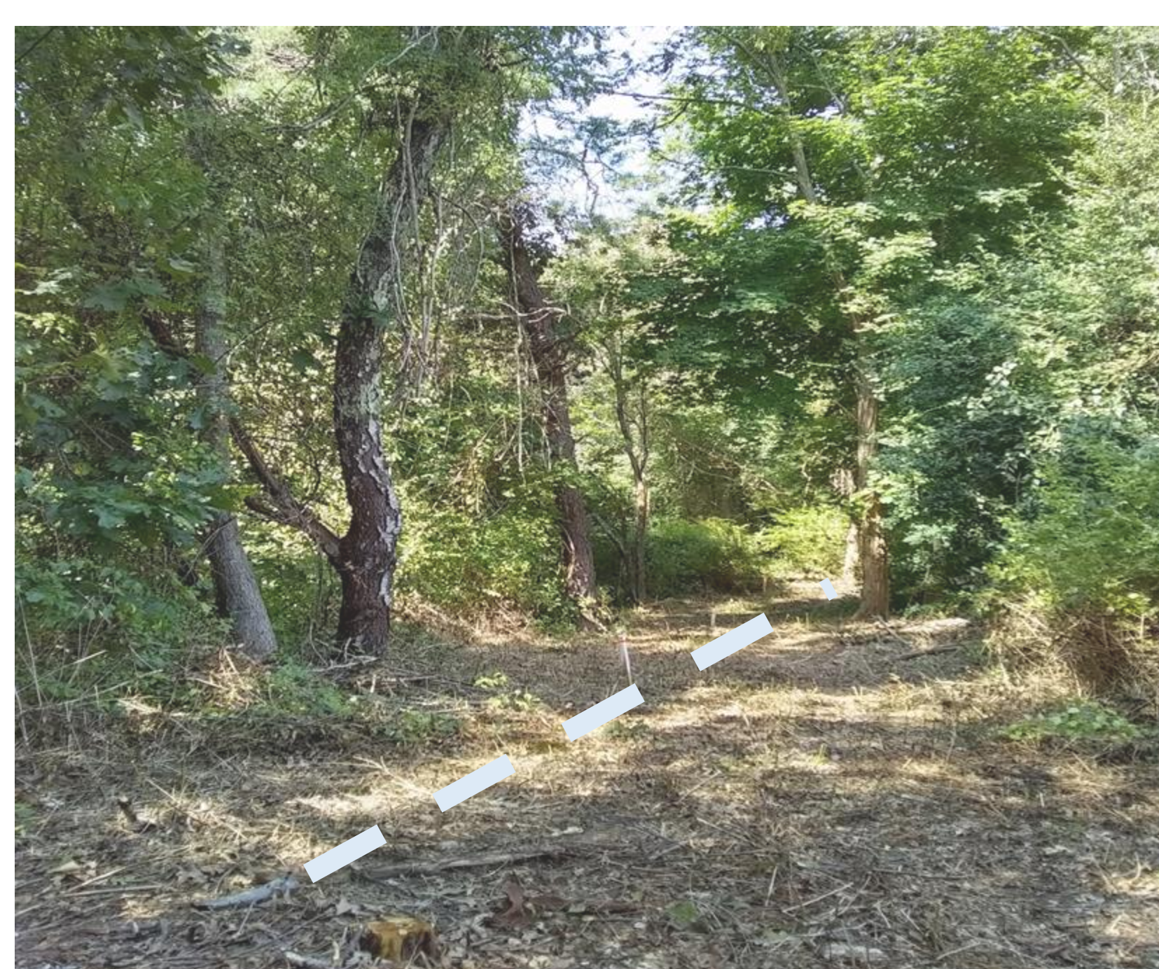
Clearing at Shorewood Drive for the PRB mapping. Clearing will not remove any mature trees, only underbrush and small saplings. Pictured represents the anticipated amount of clearing required for the PRB installation.
