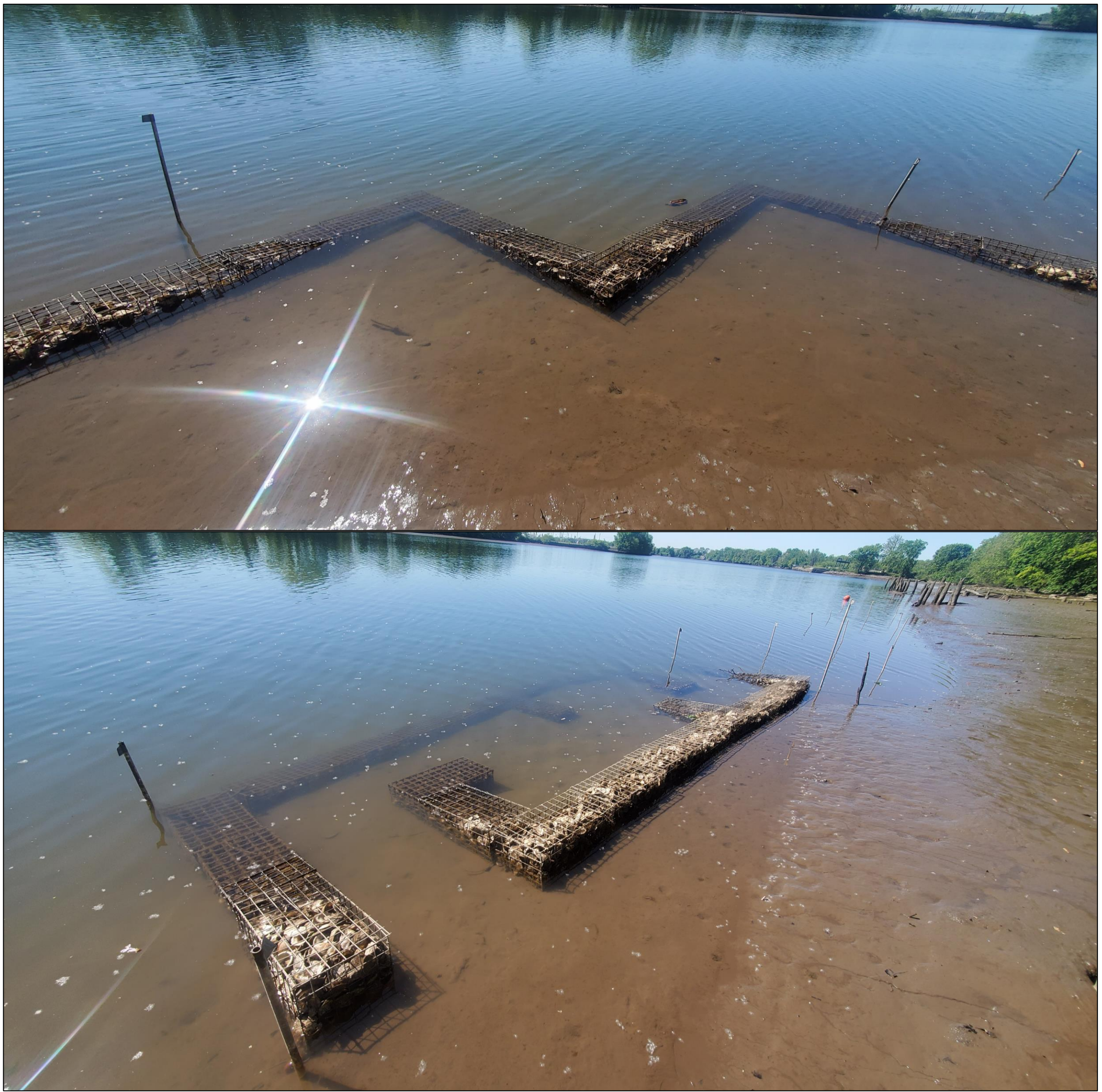
Figure 4. Image of the “W” (top) and “G” (bottom) shaped living shoreline structures at Bartram’s Garden.
