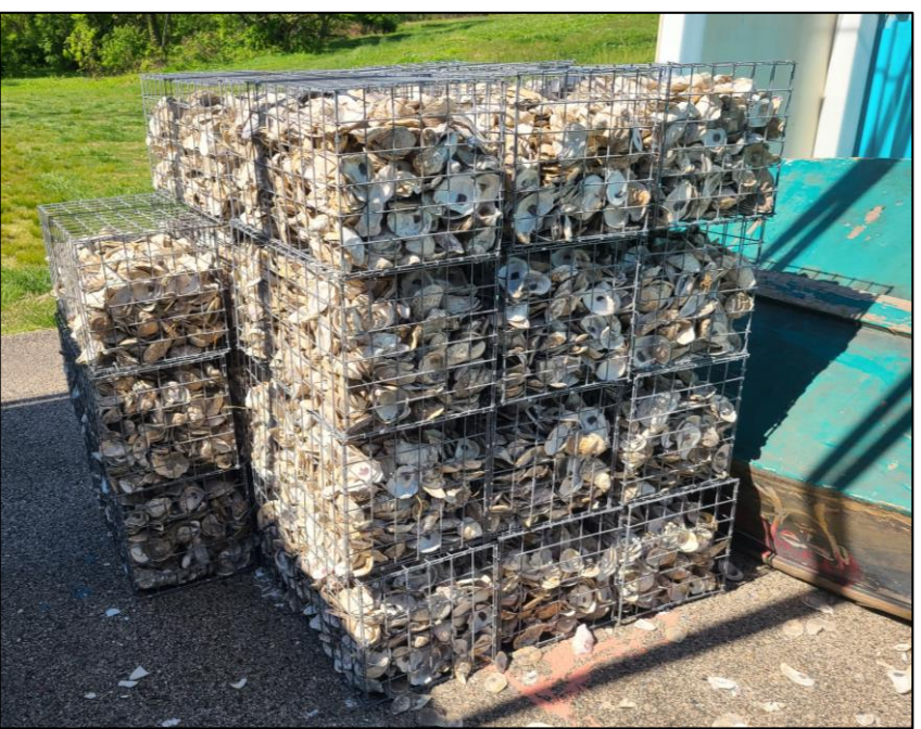
Figure 2. Gabion structures filled with recycled oyster shell.
