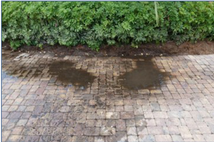
Ponding (more than an hour after rain) – Restore infiltration
