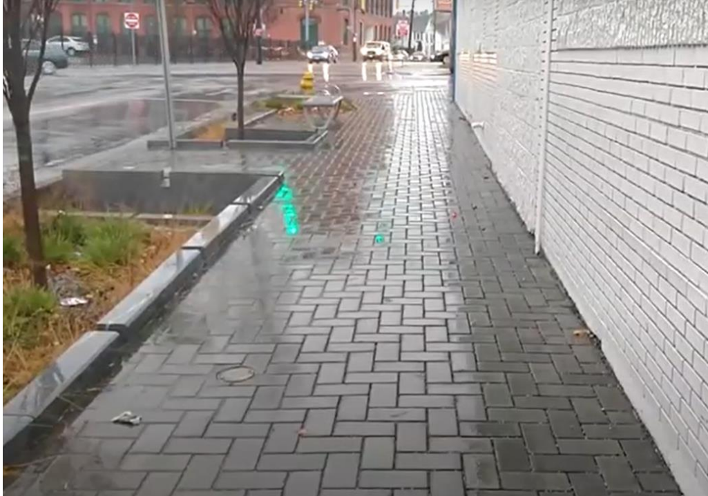
Figure 5. Pervious paver sidewalk
