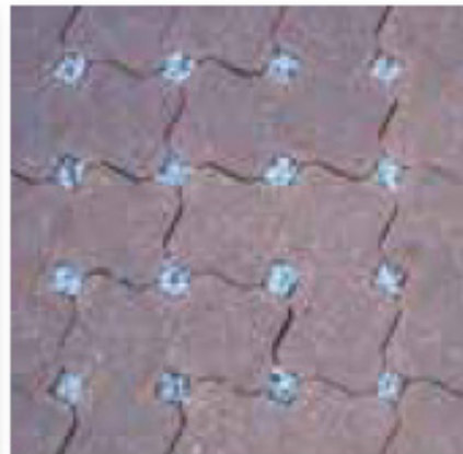
Covered joint material – Normal maintenance and replenish joint material
