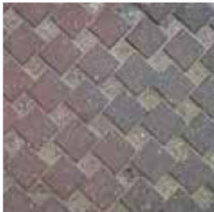
Covered joint material – Normal maintenance and replenish joint material
