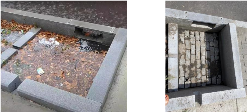
Figure 3. Grouted forebays, in use and after being cleaned.
