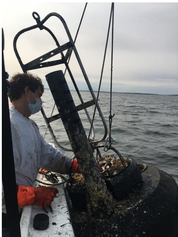
Figure 7. Work being done in 2020 to Conimicut Point buoy to re-install counterweight with added security measures - such as adding a cable around cage counterweight, so if bolts fail, the counterweight will not drop off the buoy.
