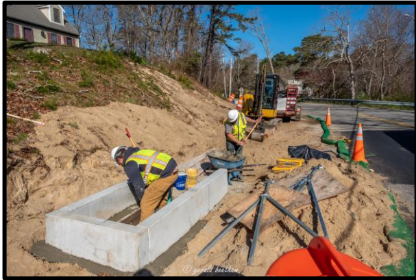
A series of three small swales were constructed in the narrow right-of-way to capture and treat runoff before flowing into the Marstons Mills River.
