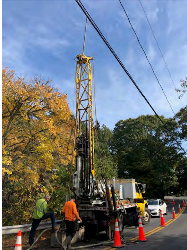
Figure 7 Soil Boring Tighe & Bond
