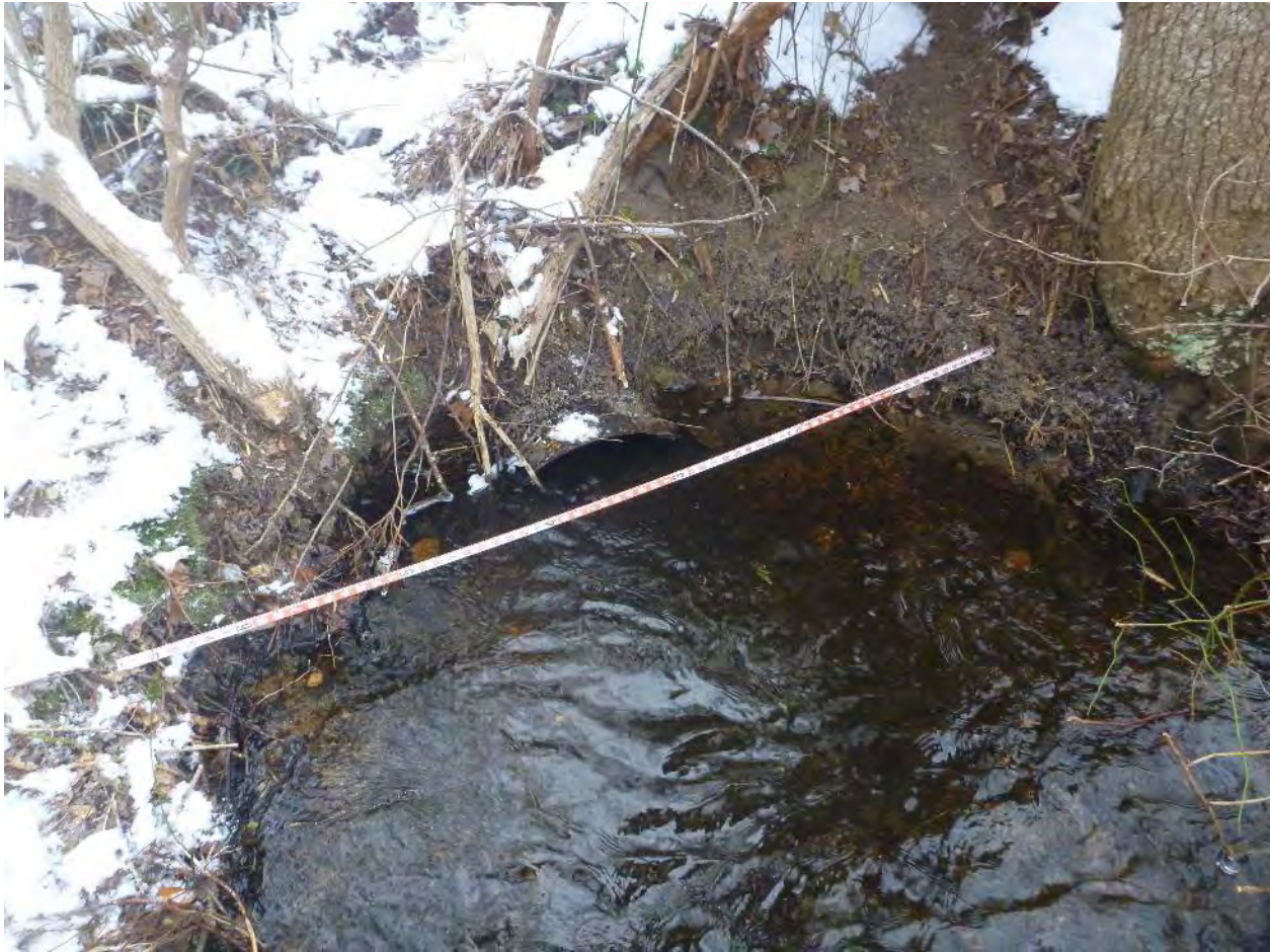
Figure 8. Looking upstream at the 18-inch corrugated metal pipe under the earthen berm and walkway between Cheyenne Lane and Knollwood Drive
