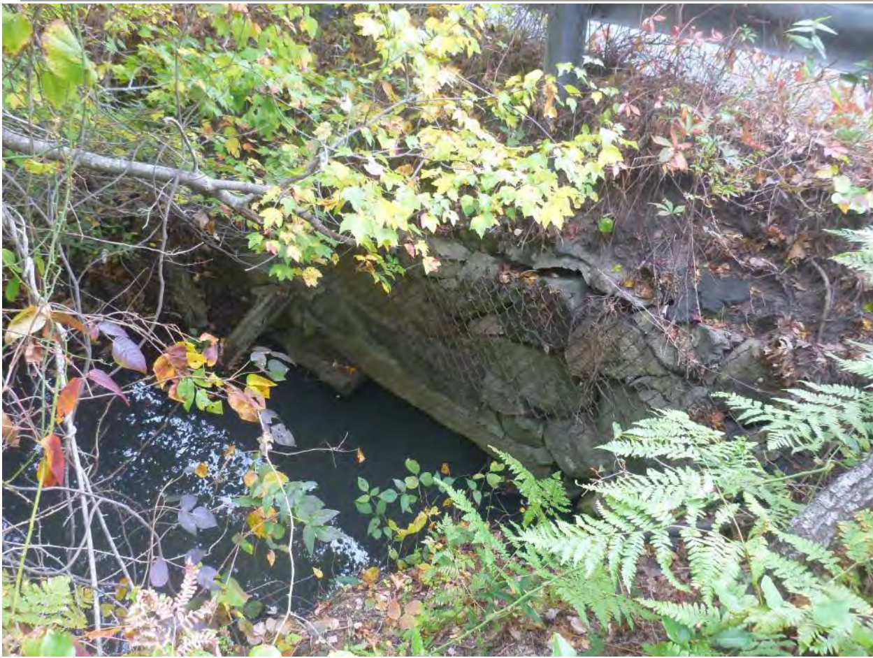
Figure 7. Culvert at Weir Road
