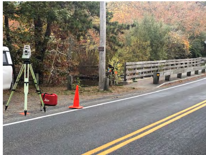
Figure 3 Culvert Survey Tighe & Bond
