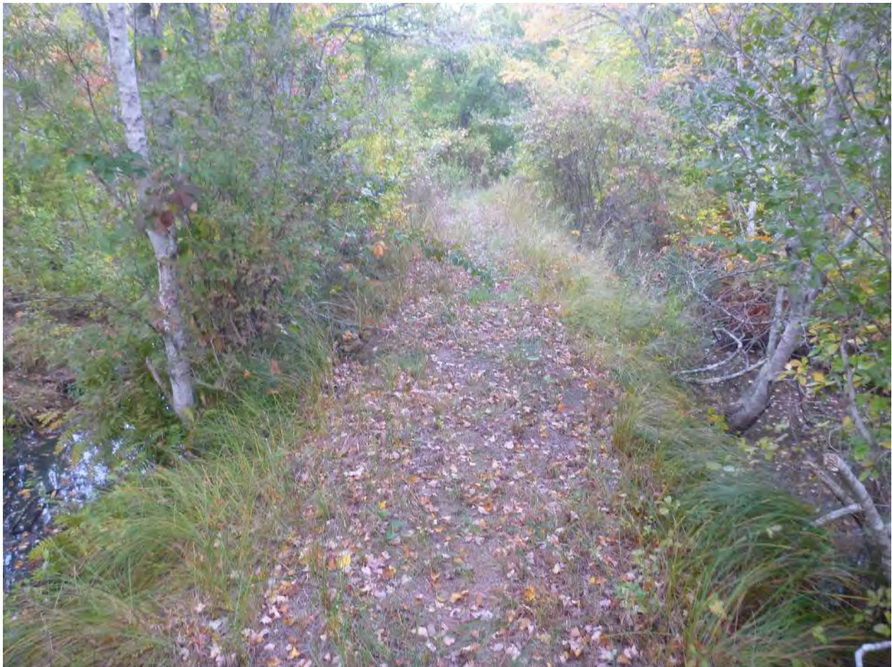
Figure 5. Looking downstream along the top of a levee separating Cells 1 & 3 from Cells 2 & 4. The main channel within the Project Site runs along the left toe of the levee in Cell 3.
