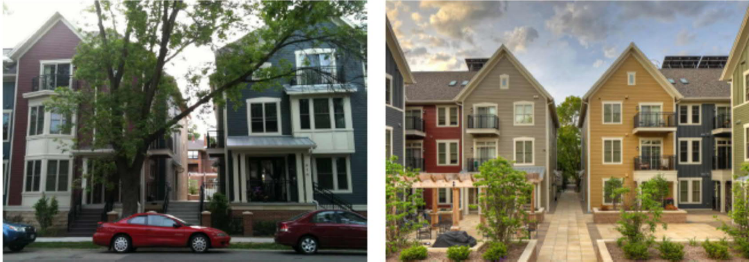
Figure 77. Multi-Family Buildings – City Row, Madison, WI
