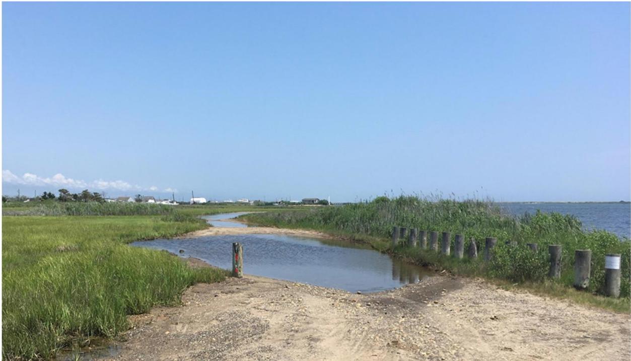
Figure 64. Image of Flooded Roadway at Mastic Beach
