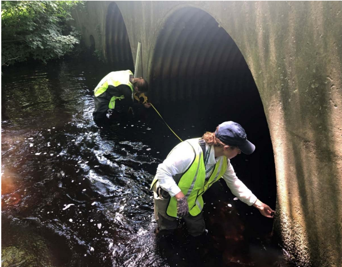
Wading in: RTWN's Helen Zincavage of SRPEDD conducts a culvert assessment for the Town of Dighton
