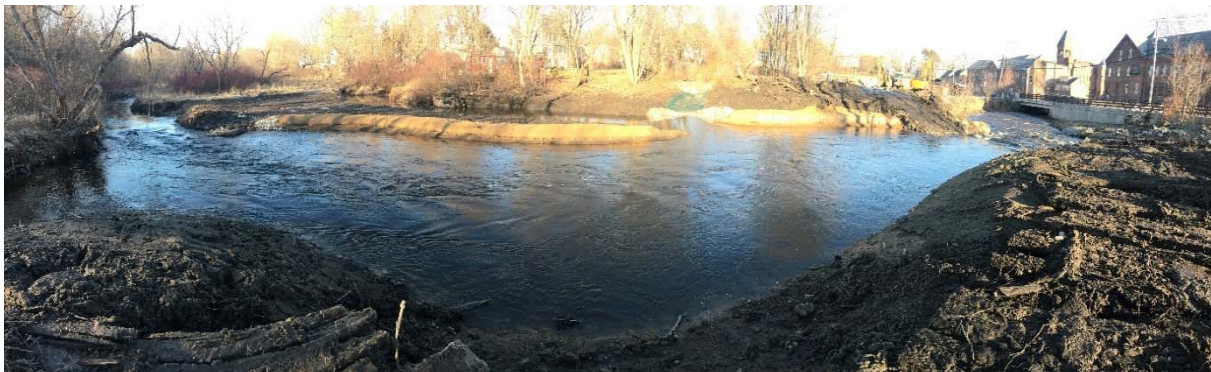
Panoramic view of the West Britannia dam removal, riverbank and parking lot restoration project in Taunton
