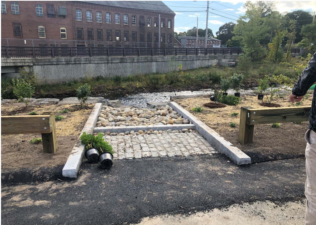
Final site restoration/reclamation work at the former Reed & Barton parking lot on the Mill River in Taunton
