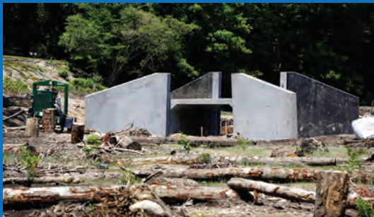
June 2021 – New Culvert in Place
