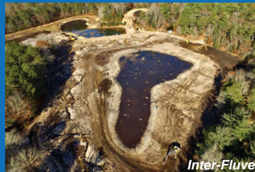
November 2020 – Ponds Completed
