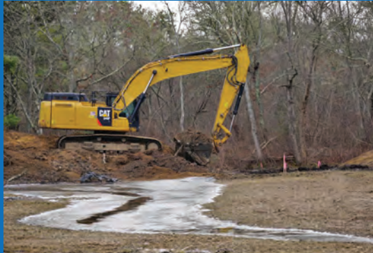
January 2021 – Dam Removal
