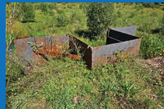
September 2018 – Bog Water Control Device Blocking Fish Passage
