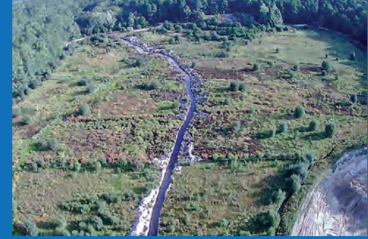
September 2020 – Diversion Channel
