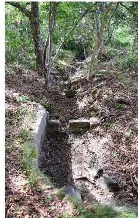
Below, 1968–2020 fish ladder, looking south from north end of the lateral section of the historic dam.
