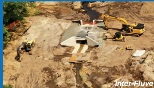
June 2021 – Construction of New Road
