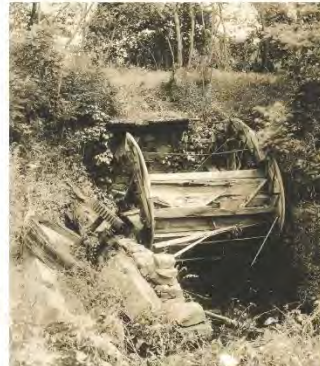
At left: Ca. 1930s photograph of the ruins of the mill's wooden waterwheel in its stone-lined pit. A part of the gear assembly used to turn the mill's machinery is on the left. (Credit: Falmouth Historical Society)
