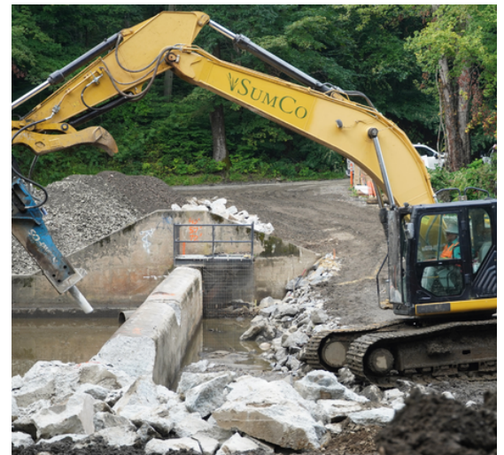
Removing Dana Dam.
