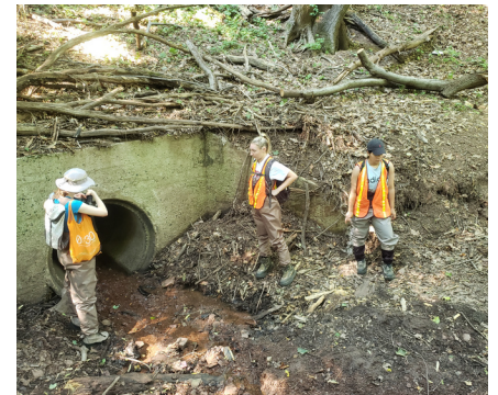
HRF staff survey a culvert in the Raritan River watershed.
