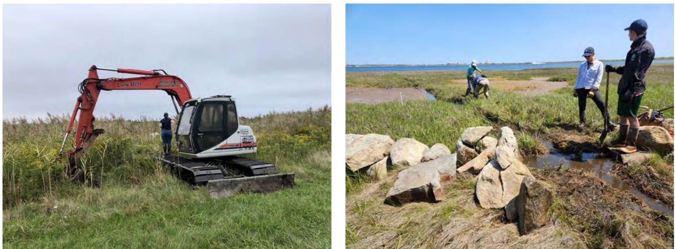
Figure 3. Large rocks (left image) and segments of submerged stone walls (right image) were removed from five key locations across Allens Pond to drain ponding water and to restore tidal hydrology to areas along the marsh/upland boundary.
