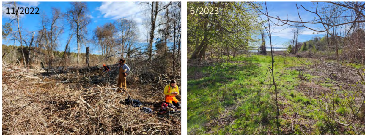
Figure 7. Mechanical brush removal was implemented to control dense, stands of invasive brush that characterized the low-lying upland areas along the saltmarsh boundary at Great Neck. The left photo was taken during brush removal and the right photo shows the area after brush removal, follow up control treatments and seeding with native grasses.
