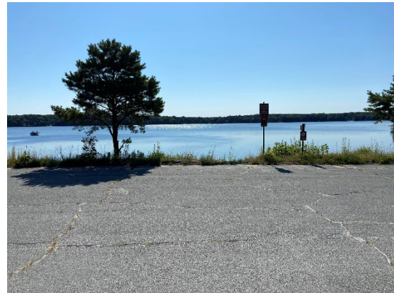
Figure 4: Ashumet Pond Boat Ramp parking lot looking east. Photo credit: APCC.
