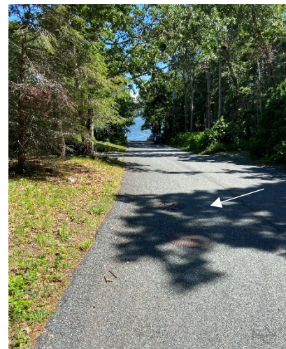
Figure 8: Follins Pond Road Boat Ramp in Yarmouth. Arrow indicates existing catch basin. Photo credit: APCC.
