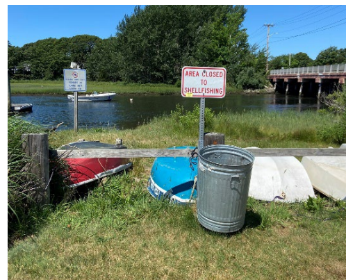
Figure 10: Photo taken from Herring River Boat Ramp showing the Route 28 bridge under which the secondary water main pipe will be drilled. Photo credit: APCC.
