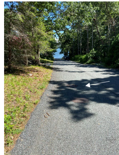
Figure 8: Follins Pond Road Boat Ramp in Yarmouth. Arrow indicates existing catch basin. Photo credit: APCC.
