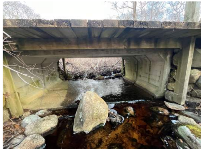
Image 3. Wooden Vehicle Crossing Downstream Culvert (March 19, 2024)
