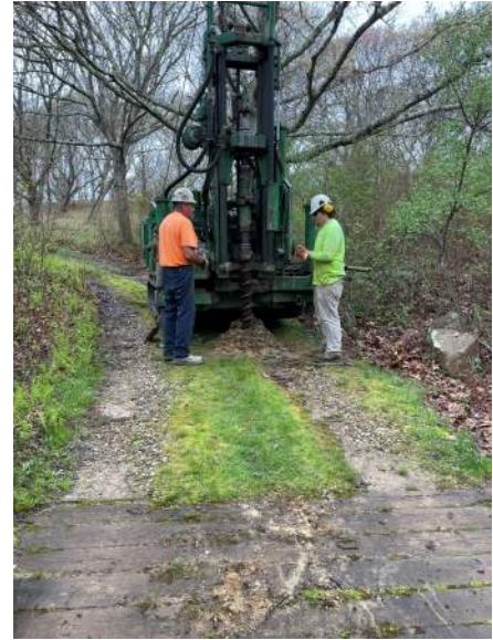
Image 8. Wooden Vehicle Crossing Soil Boring
