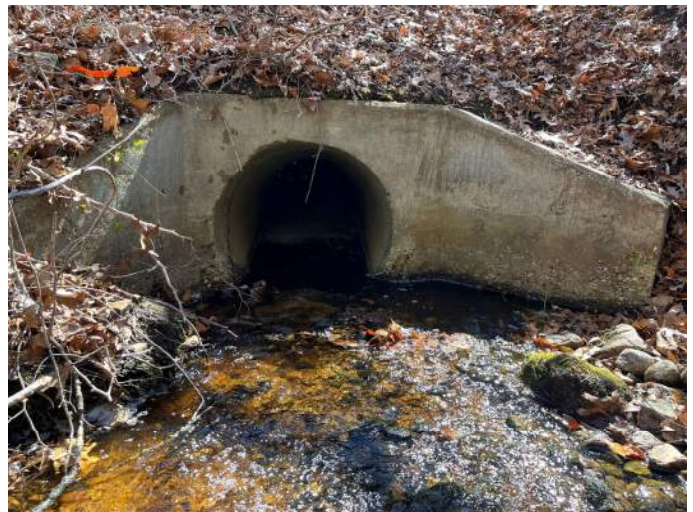
Image 2. Moshup Trail Crossing Upstream Culvert (March 19, 2024)
