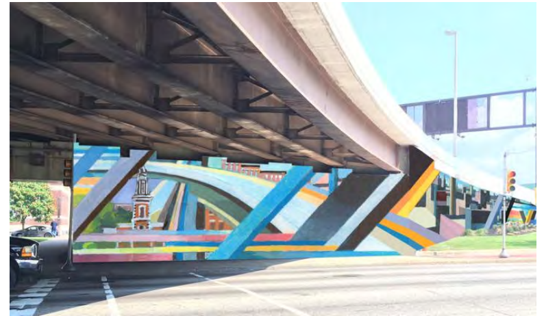
Electric Philadelphia Mural & Light Installation – Day (Philadelphia, PA)
