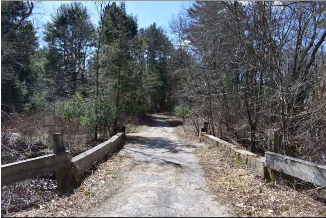
Photo 16. Concrete arch bridge deck on Burnt Sawmill Road, view south.
