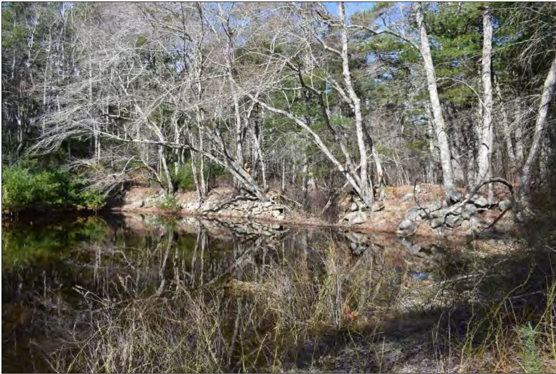
Photo 20. Sweet Pond Dam, view northwest.
