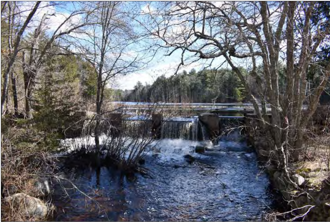
Photo 1. Capwell Mill Pond Dam, view east.
