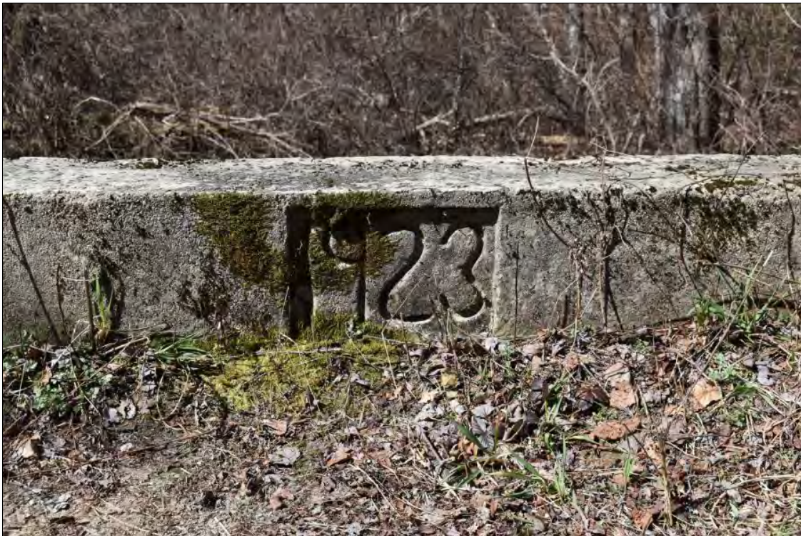
Photo 17. Engraved "1923" dedication on the concrete arch bridge, view west.
