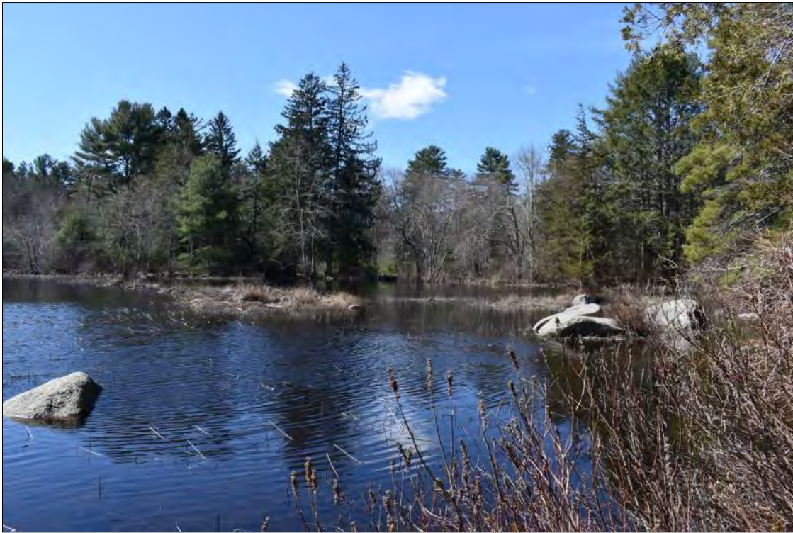
Photo 18. Legacy dam remains in Capwell Pond, view south.
