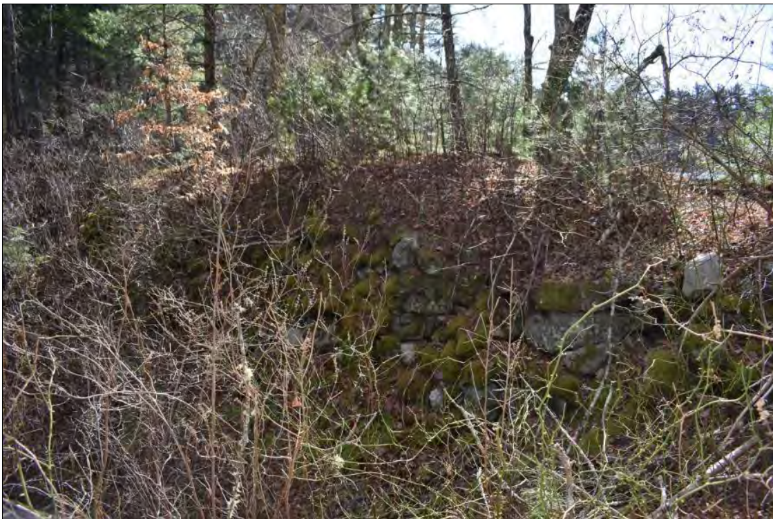
Photo 25. Downstream (north) face of the Sweet Pond Dam, view southeast.
