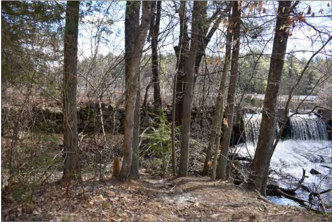
Photo 3. Downstream (west) face of the Capwell Mill Pond Dam, view east.
