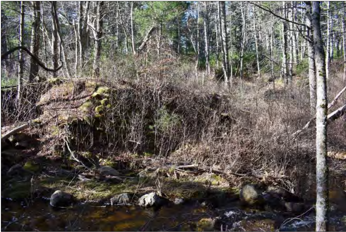
Photo 33. Sweet Pond Dam wheel pit remains, view west.
