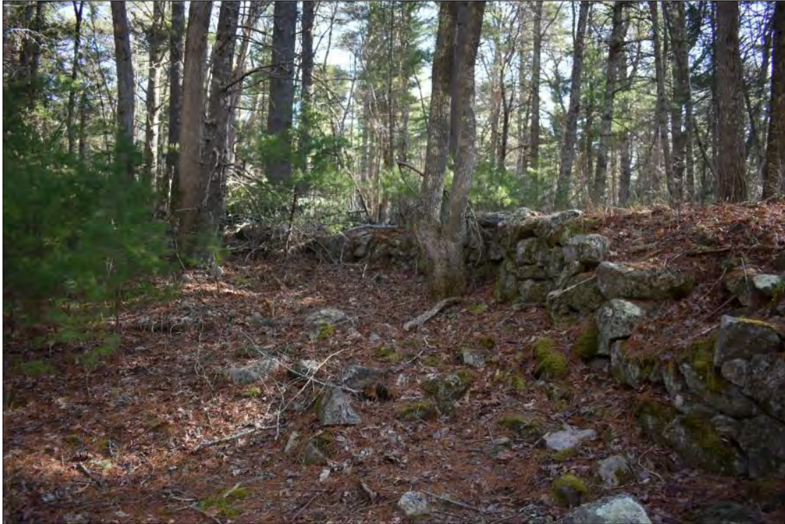
Photo 37. Sweet Pond Dam northeast abutment wall, view east.
