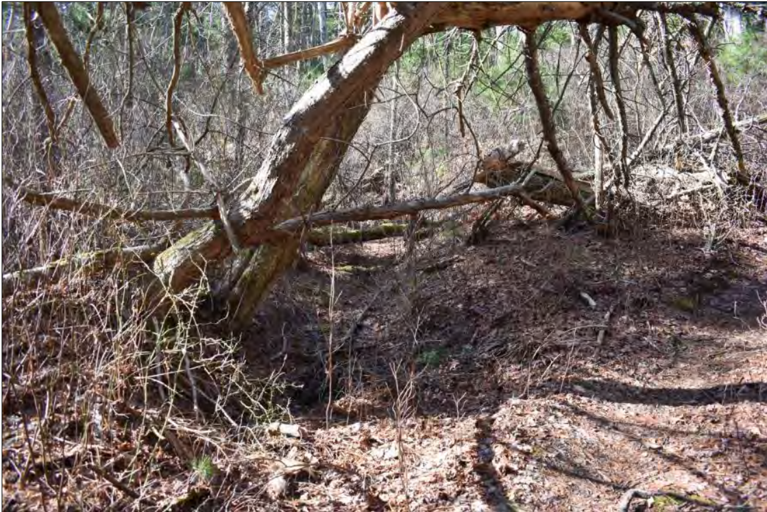
Photo 34. Sweet Pond Dam channel, view southwest.
