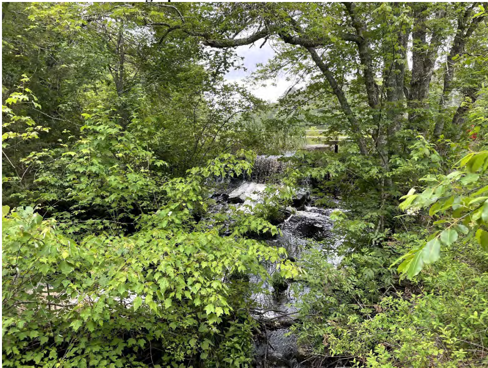
Photograph 6: View of dam from Burnt Sawmill Road.
