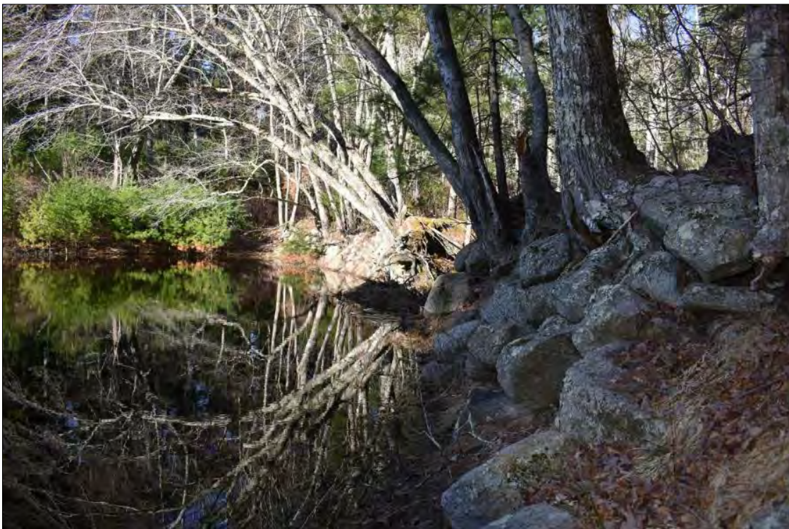
Photo 23. Upstream (south) face of the Sweet Pond Dam, view west.
