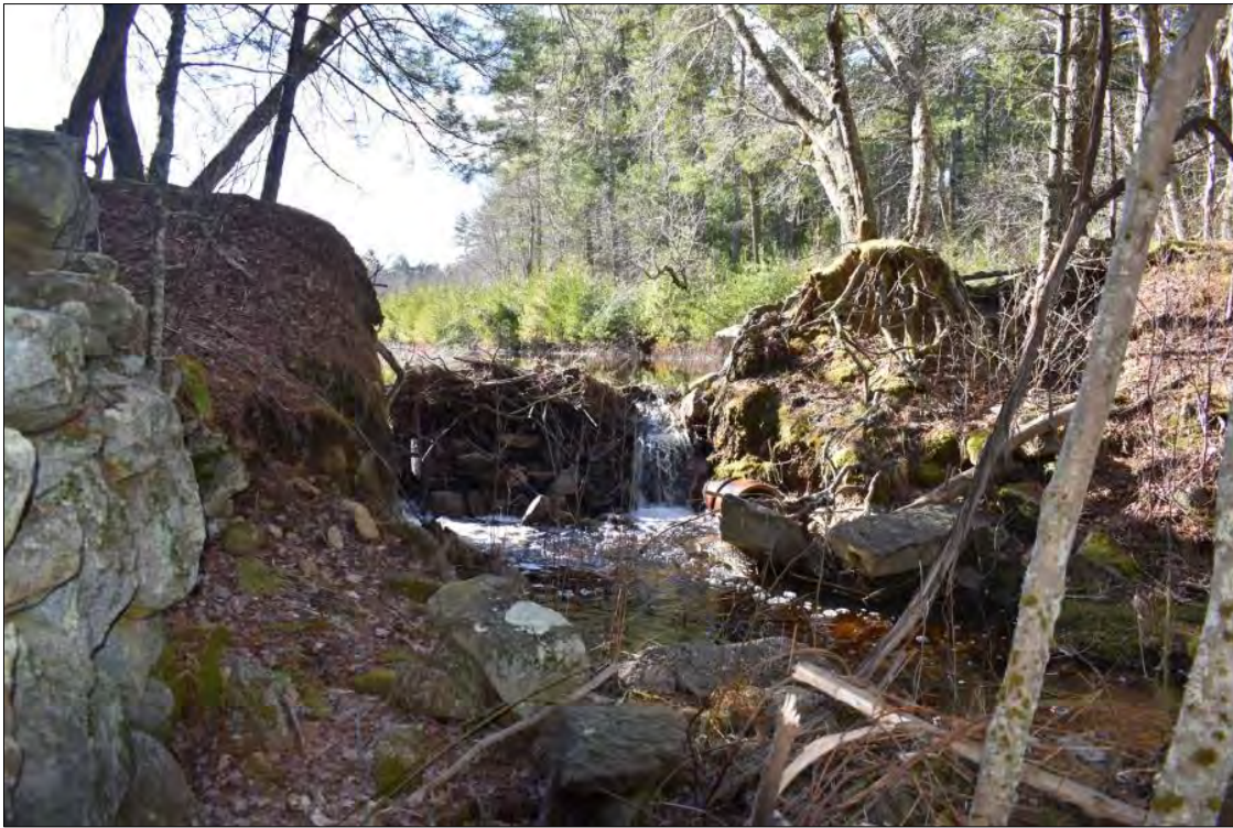
Photo 31. Sweet Pond Dam spillway, view southwest.
