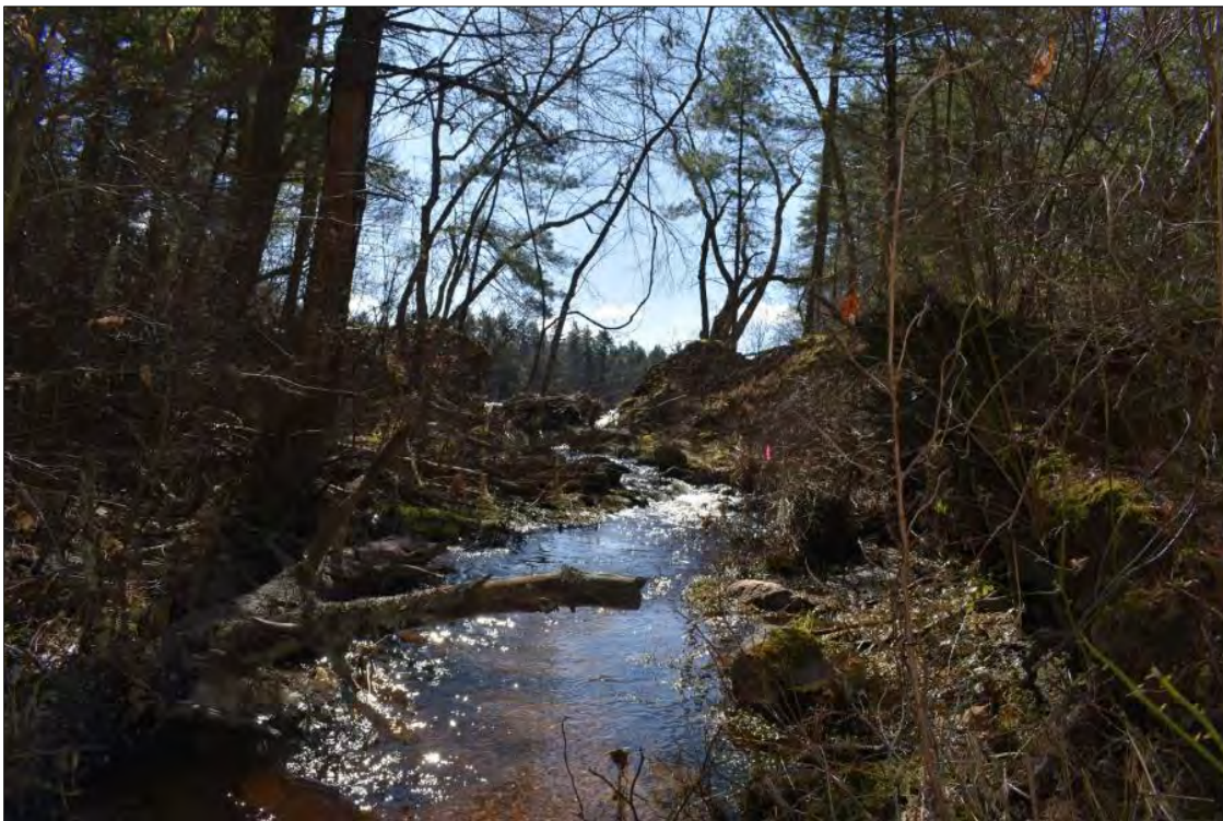
Photo 30. Sweet Pond Dam spillway and upstream reach, view south.
