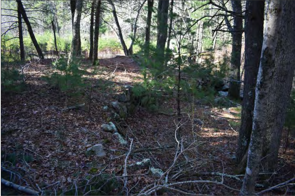
Photo 27. Downstream (north) face of the Sweet Pond Dam, view west.
