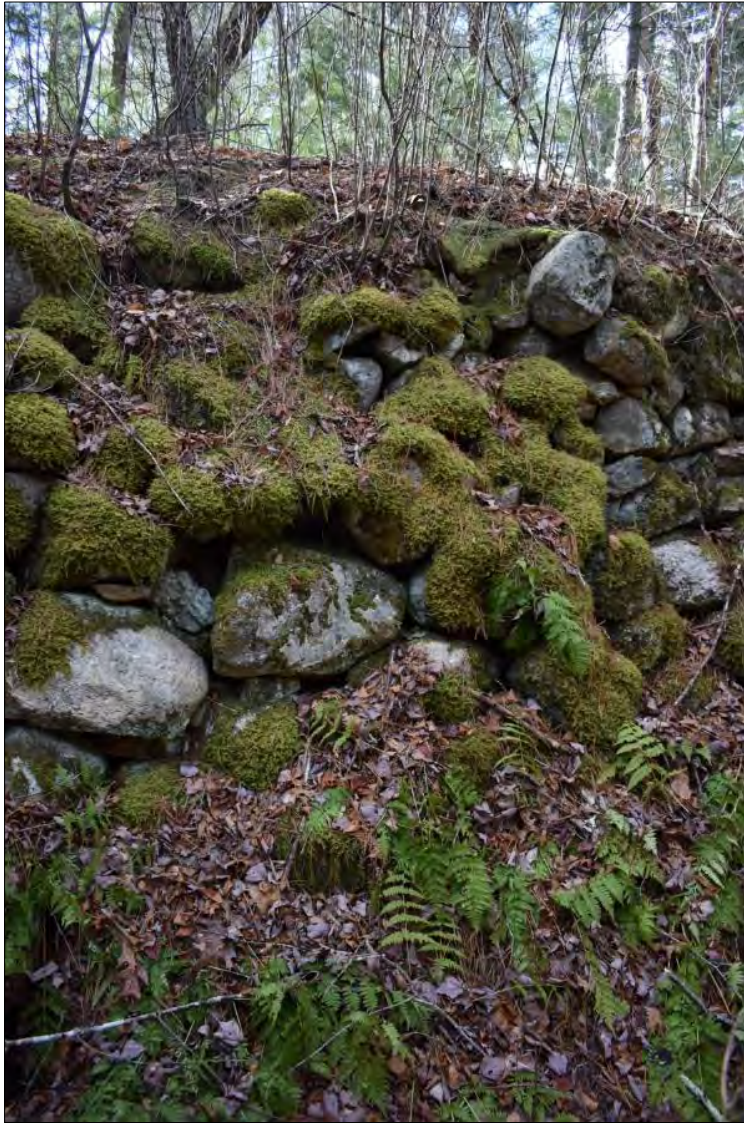
Photo 26. Downstream (north) face of the Sweet Pond Dam, view south.
