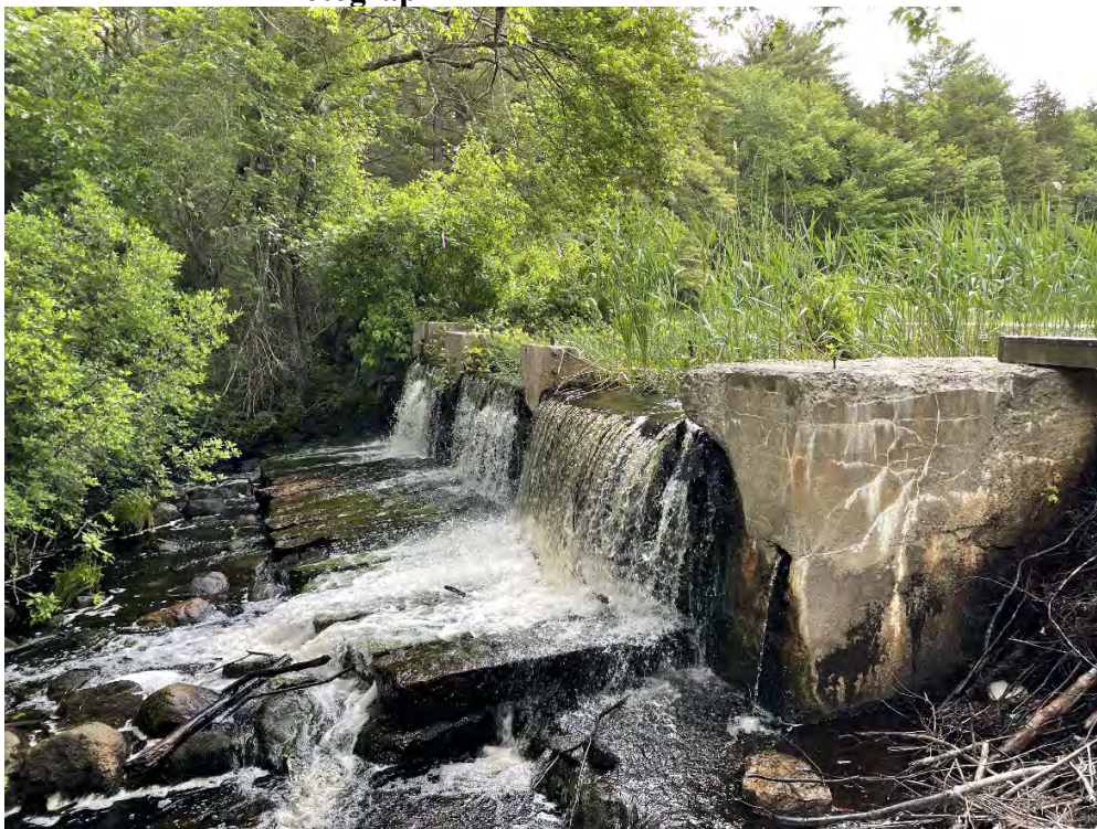
Photograph 8: Main dam area.
