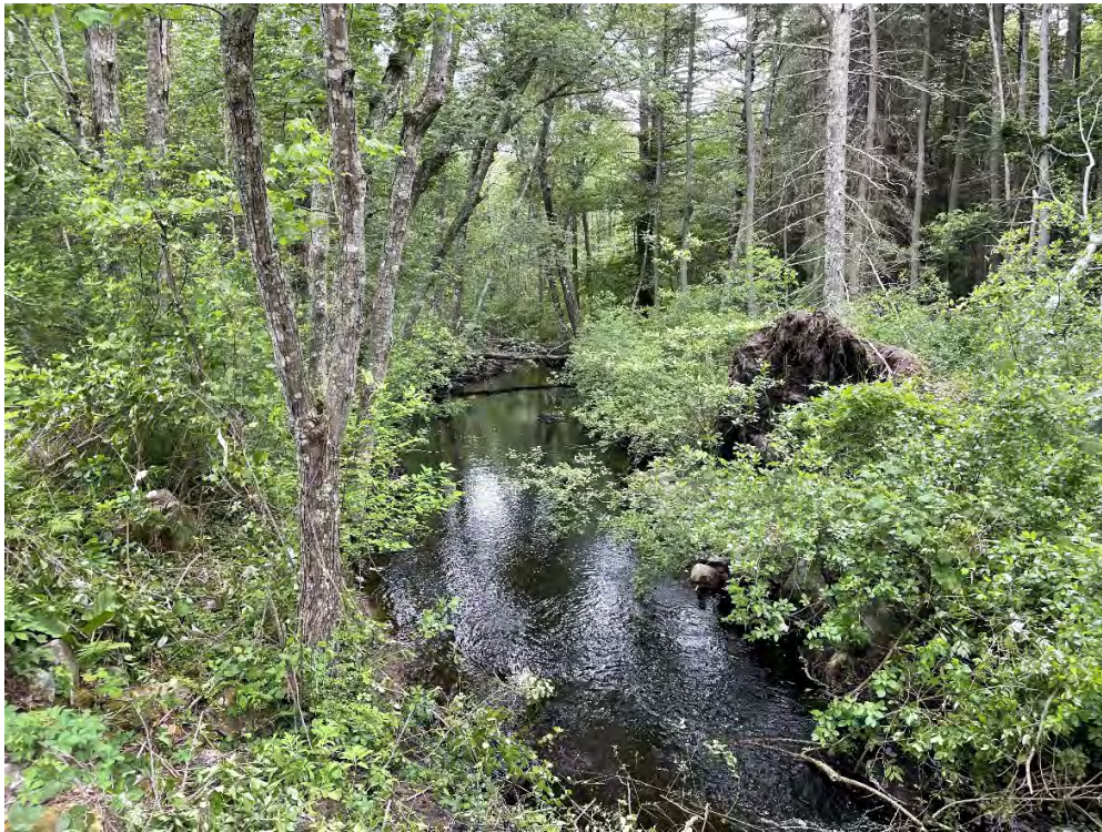
Photograph 7: View downstream of dam.
