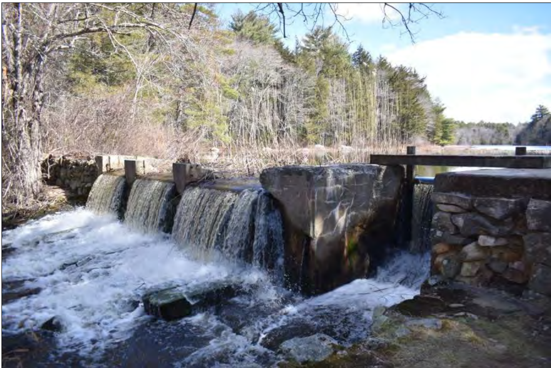
Photo 10. Capwell Mill Pond Dam spillway and sluice, view northeast.
