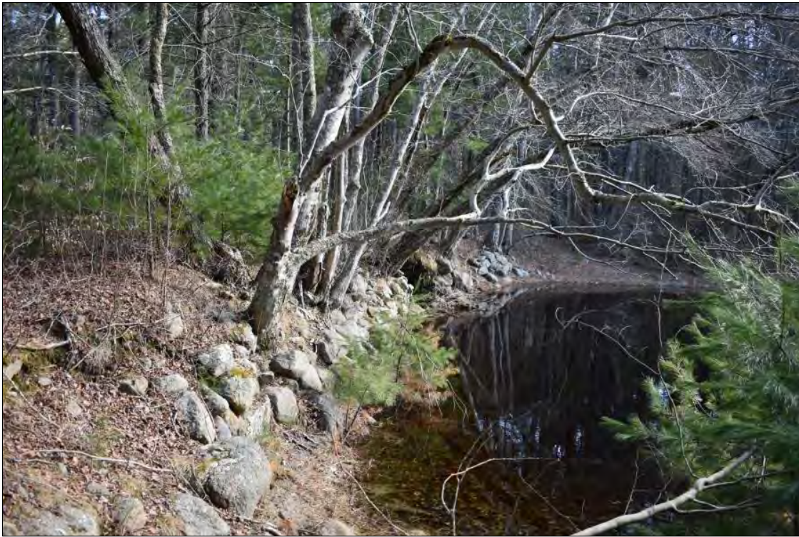
Photo 24. Upstream (south) face of the Sweet Pond Dam, view east.
