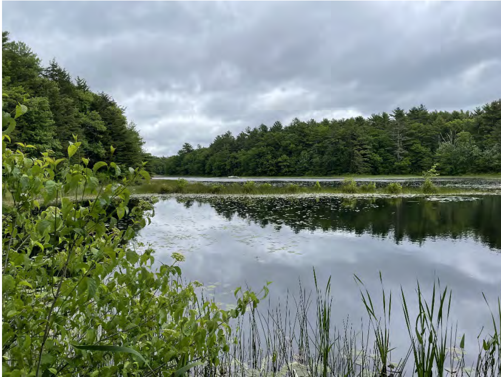
Photograph 5: View from south side of dam.
