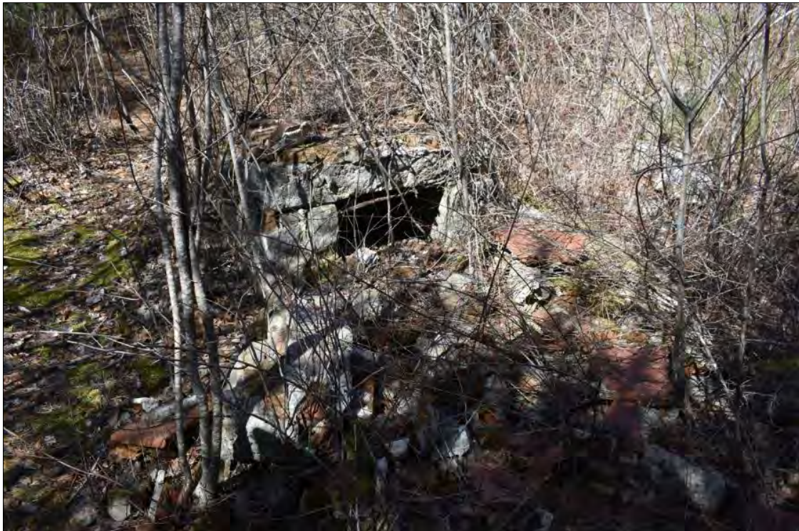
Photo 19. Concrete and brick pad to the southeast of the Capwell Mill Pond Dam, view west.
