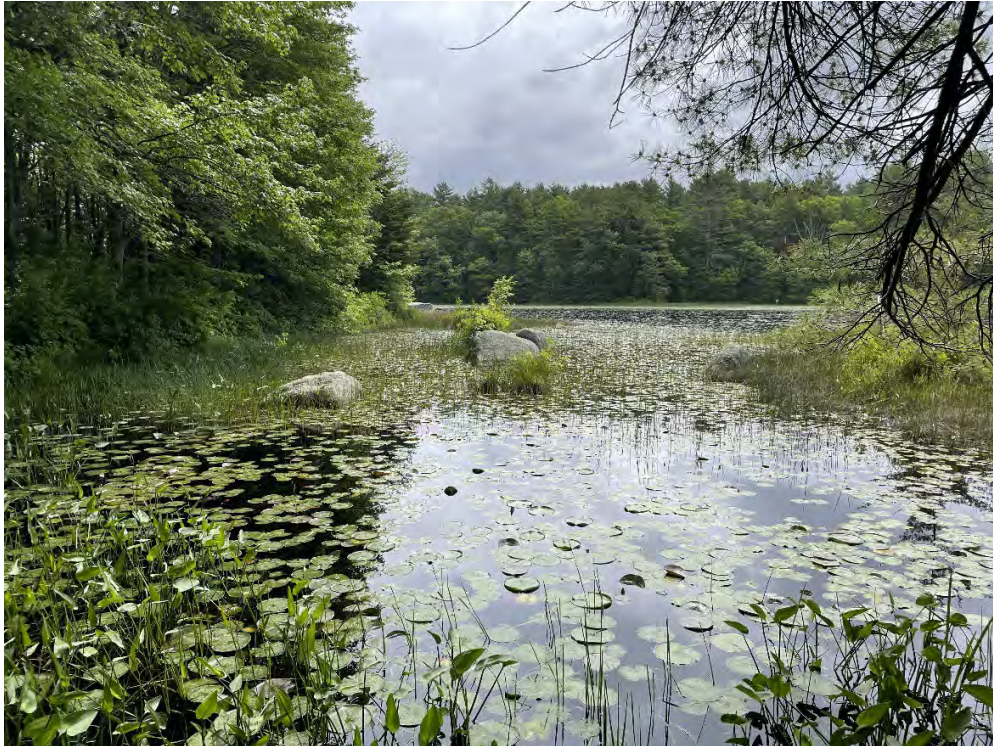
Photograph 4: Facing east from top of dam.
