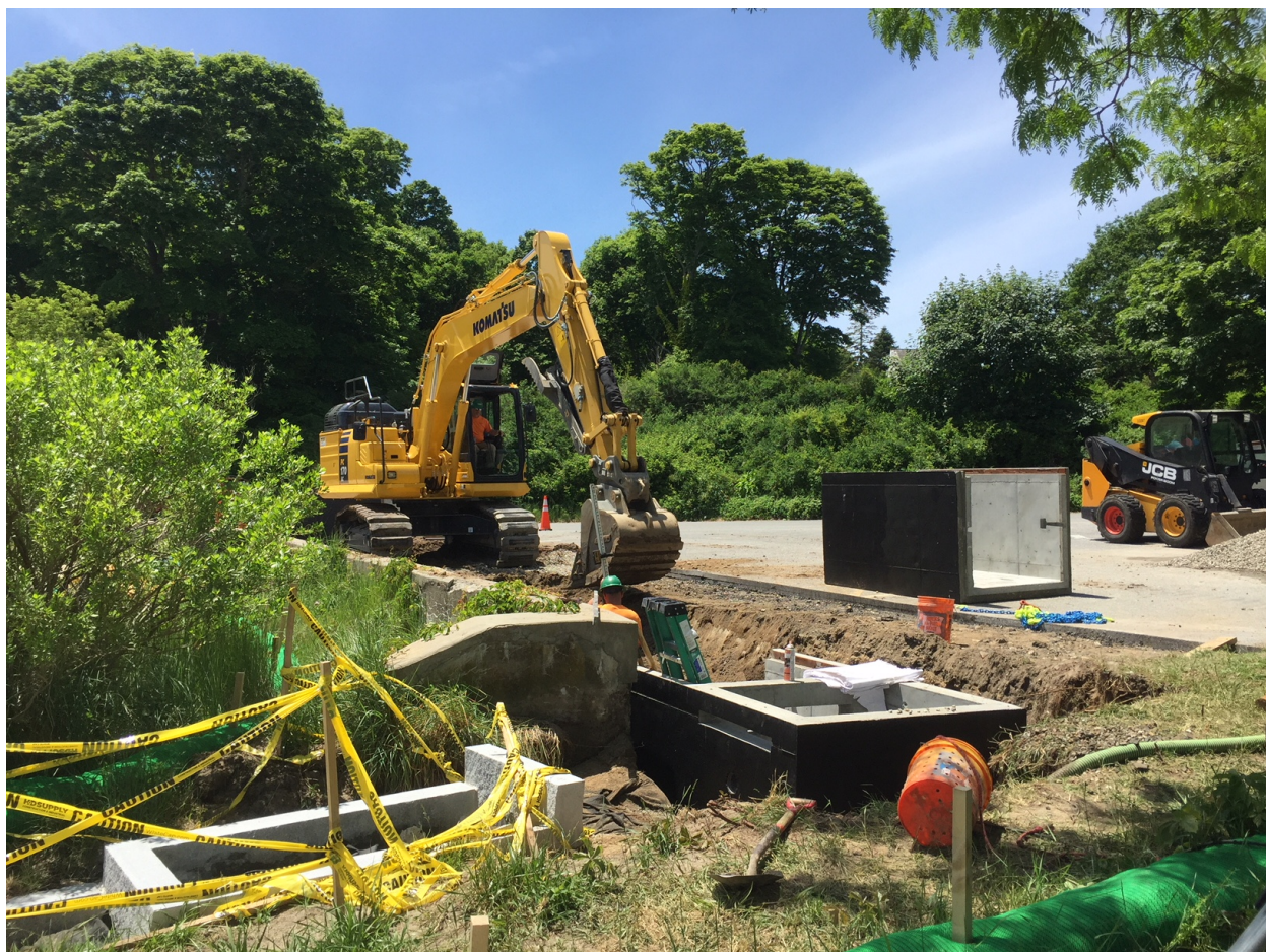
Installing a SNEP-funded stormwater infiltration system on Cape Cod.
