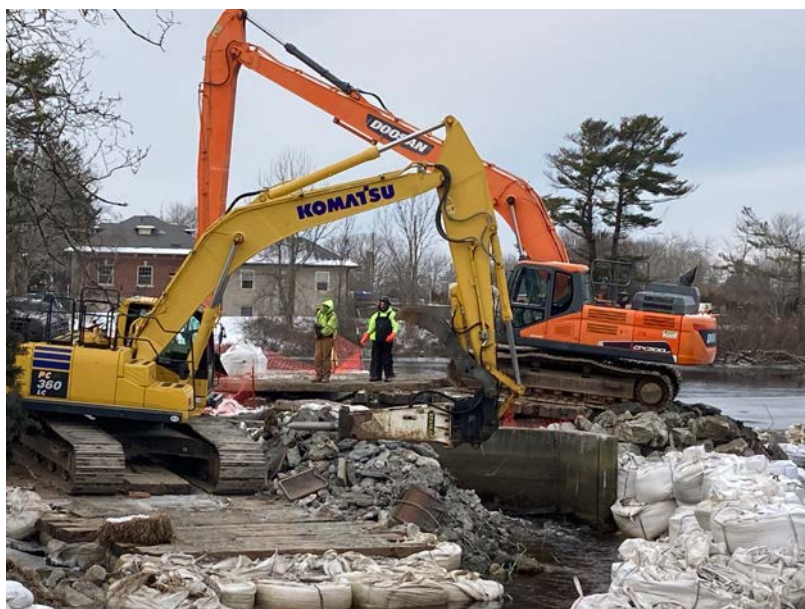
Removing Kickemuit Lower Dam.
