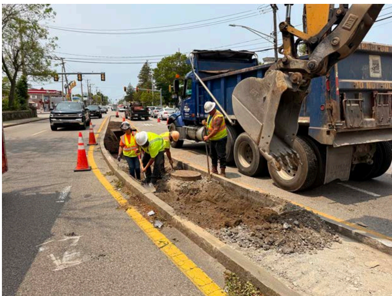
Installing stormwater measures along Kempton Avenue. Photo courtesy Green International.
